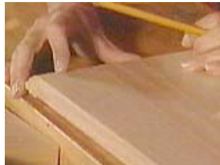
Check the cut against the base for accuracy
