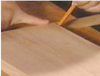
Hold the panel molding in place and mark for cutting
